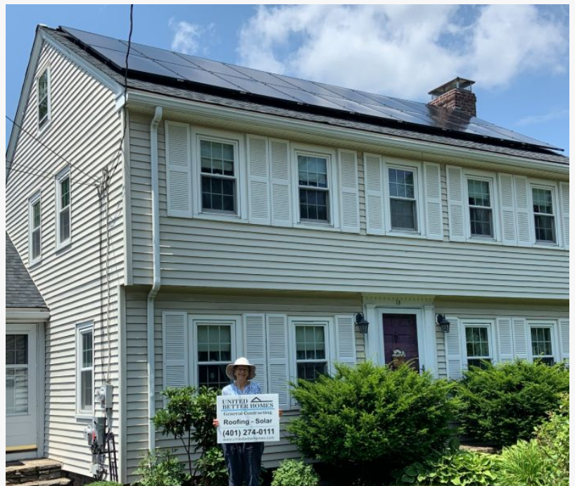
solar installation for a homeowner in Rhode Island
