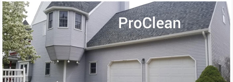
before and after power washing a home in Lansing, MI
