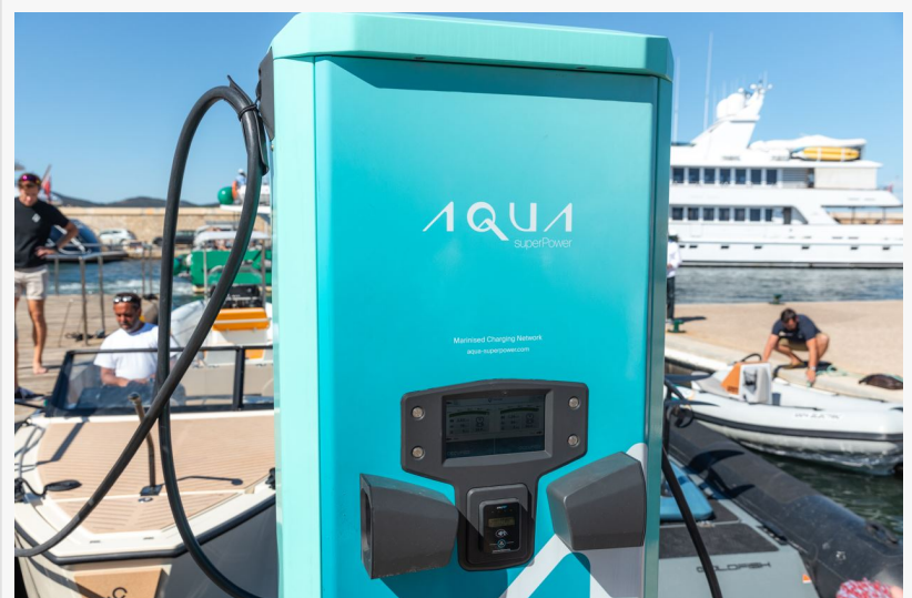
The Aqua 75 dual CCS configuration at Port de Saint-Tropez supercharging 2 electric boats simultaneously
