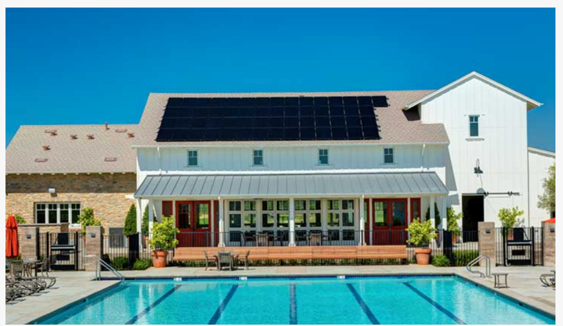
SunRev Installation with Pool
