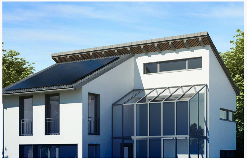
SunRev Residential Installation
