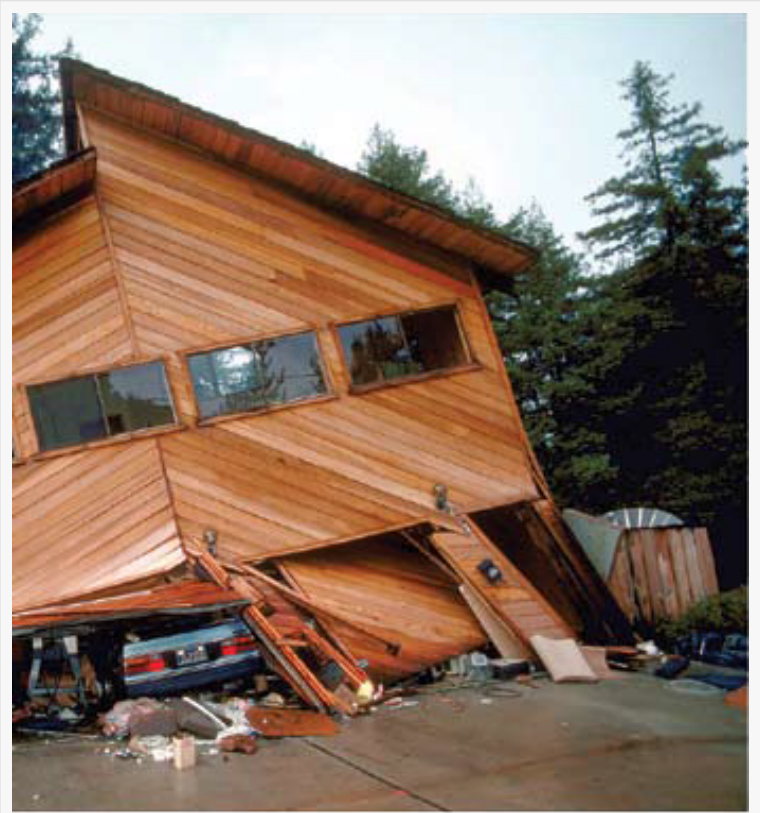
foundation repair in LA
