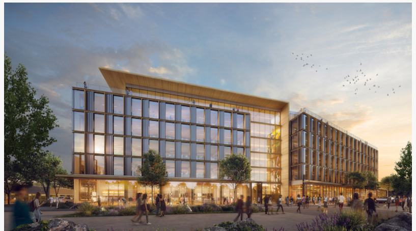
Exterior rendering of Maine's first commercial office building using primarily mass timber construction, specifically cross-laminated timber (CLT).
