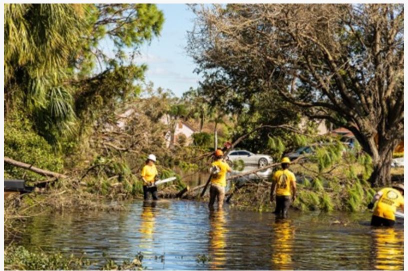
Chainsaw team clearing roads near city of Ft. Myers
