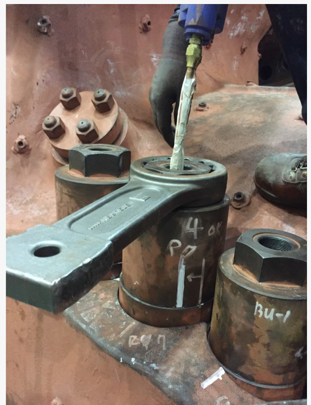
Thermo Intl. - Induction Bolt Heating Project
