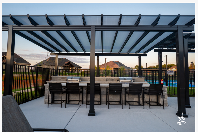
Mansfield Reserve Outdoor Pergola Covering - Selah Pools, Renaissance Patio Products
