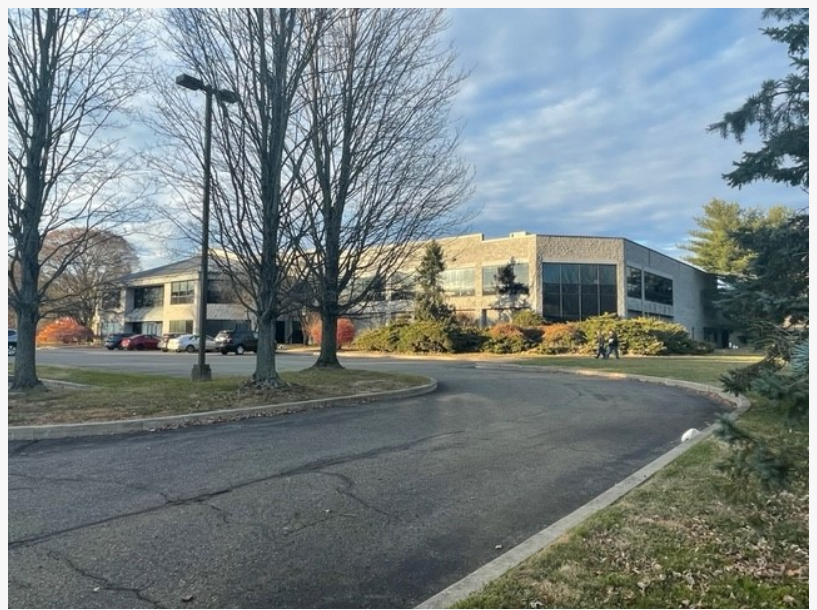
M. Davis Kennett Square Offices & Fabrication Facility
