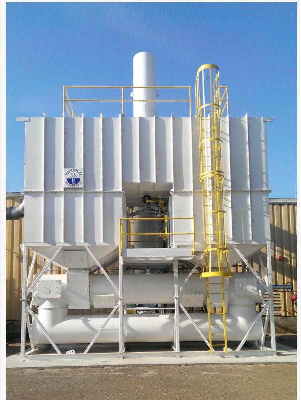
Regenerative Thermal Oxidizer Provided to Composites Manufacturing Client
