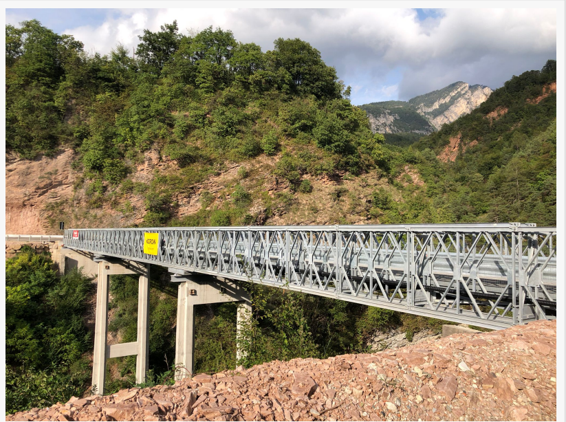
Acrow Bridge, Ton, Northern Italy
