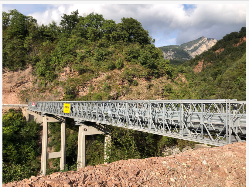
Acrow Bridge, Ton, Northern Italy
