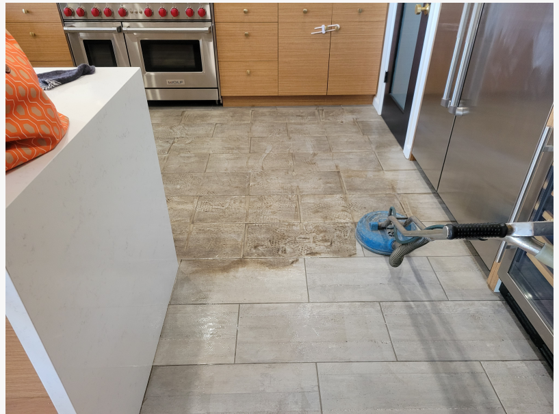
Tile and grout cleaning
