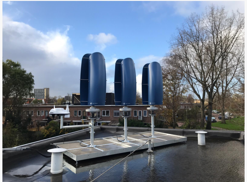
Flower Turbines Small Size Wind Tulip Installation
