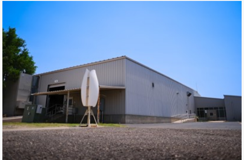
Flower Turbines Outside Manufacturing plant
