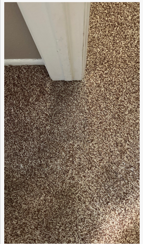
Carpet repair can remove damage caused by pets.
