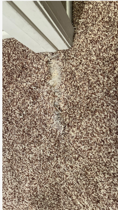
Carpet damage caused by a pet in a doorway.
