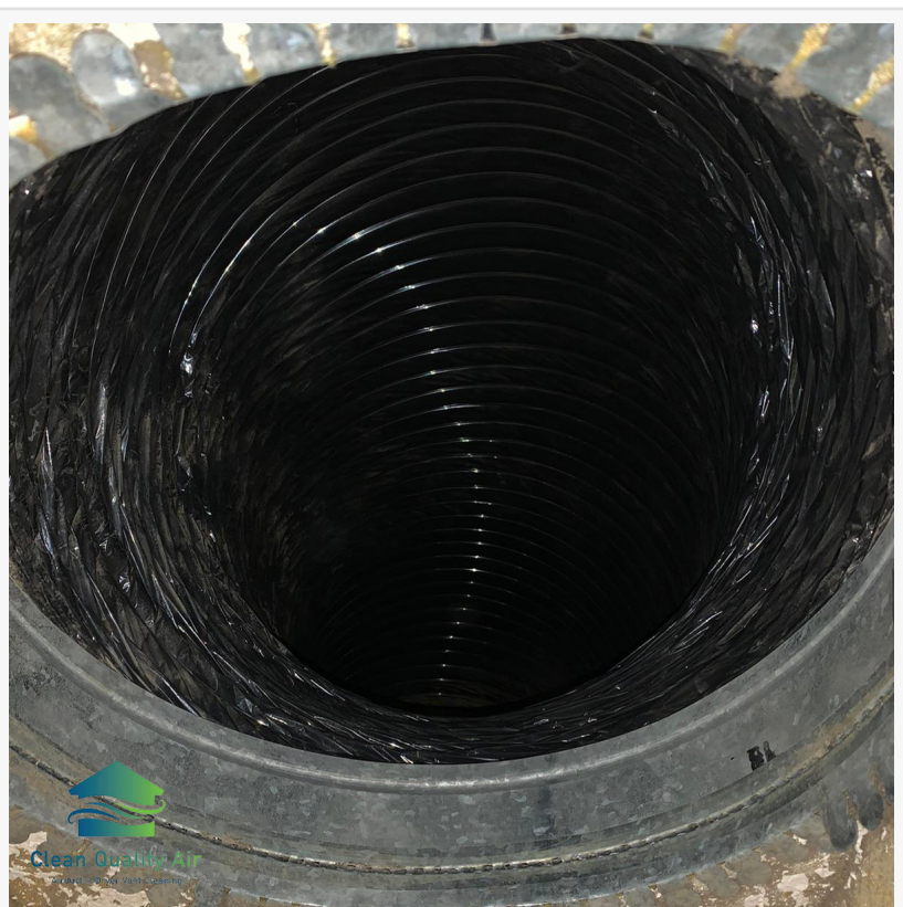
Air Duct Cleaning Services
