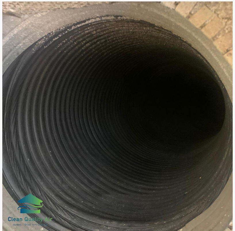
Clean Quality Air - Air Duct Cleaning
