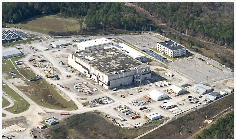
Partially finished plutonium fuel (MOX) plant at the Savannah River Site, which DOE has proposed to convert into the SRS pit plant, at a current cost estimate of $11 billion.. Photo ©High Flyer, 2020.
