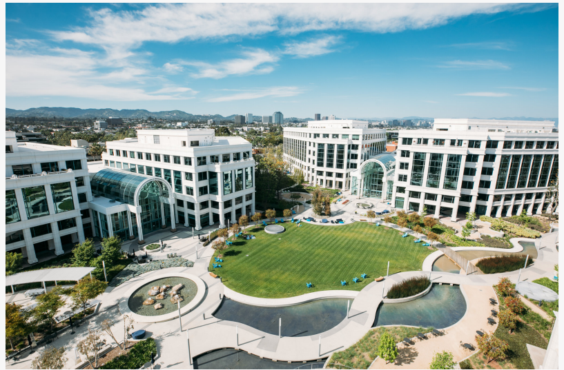
Santa Monica creative office campus Water Garden
