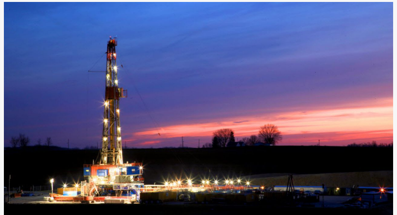
A Patterson- UTI rig drilling a well in Carroll county, OH.
