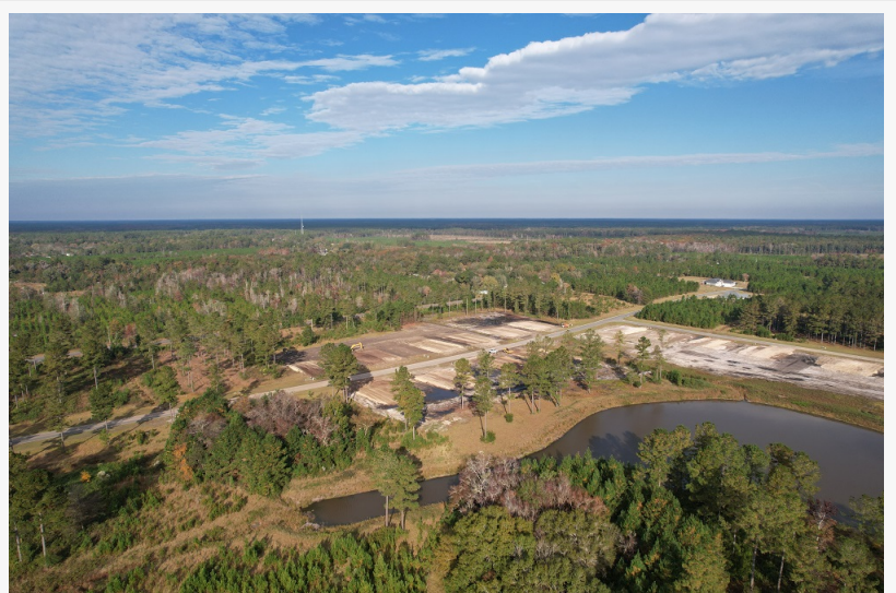
Homes under construction at Northshore
