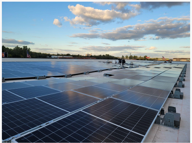
Ballast Mounted Commercial Building Solar Array
