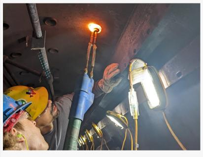
Weinacker continues, "We simplified the boiler tube removal by utilizing our portable induction machine with a specially designed internal coil. This heated the tube rapidly where it is rolled into the tube sheet. The tube reaches 2500F degrees within 30-90 seconds. This rapid heating
