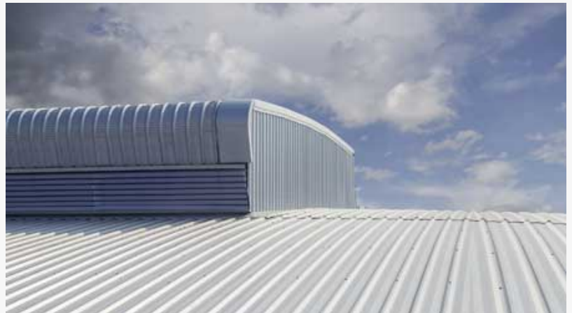
Roofing Coatings market Know The Market Driving Factors 2022
