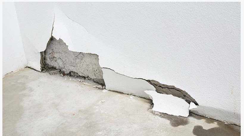
best foundation repair company in San Antonio Texas
