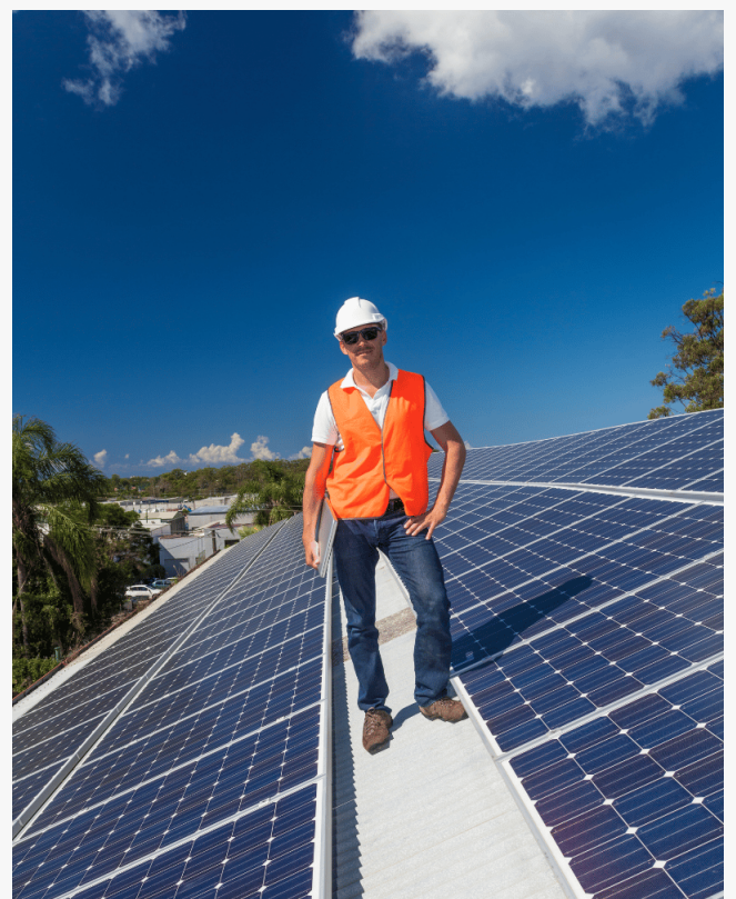
Eddie McLaughlin and commercial solar installers in Orange County help businesses save money
