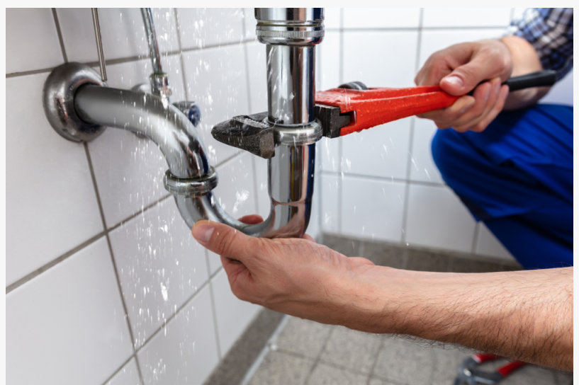
Blocked Drain Pipes
