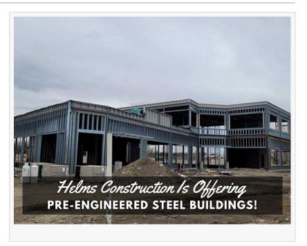
are steel structures composed of primary and secondary members, roof and wall sheeting connected, and various other building components.
