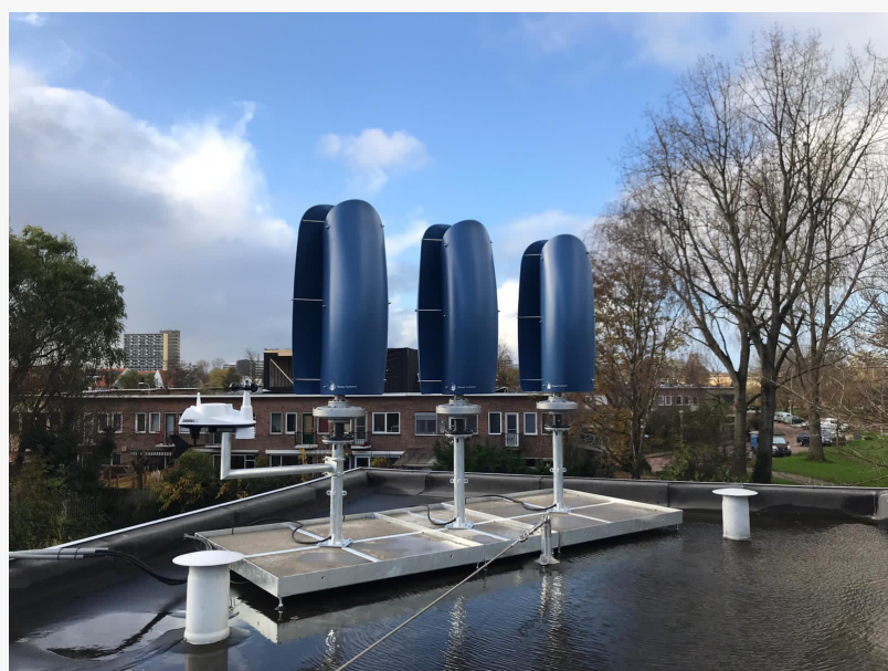
Three installed small size Wind Tulips
