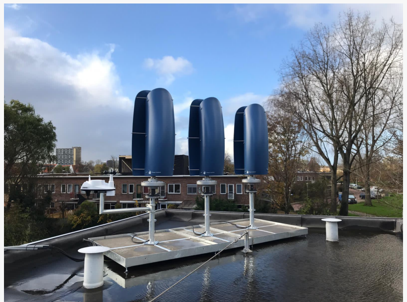
Flower Turbines Small Size Wind Tulip Installation
