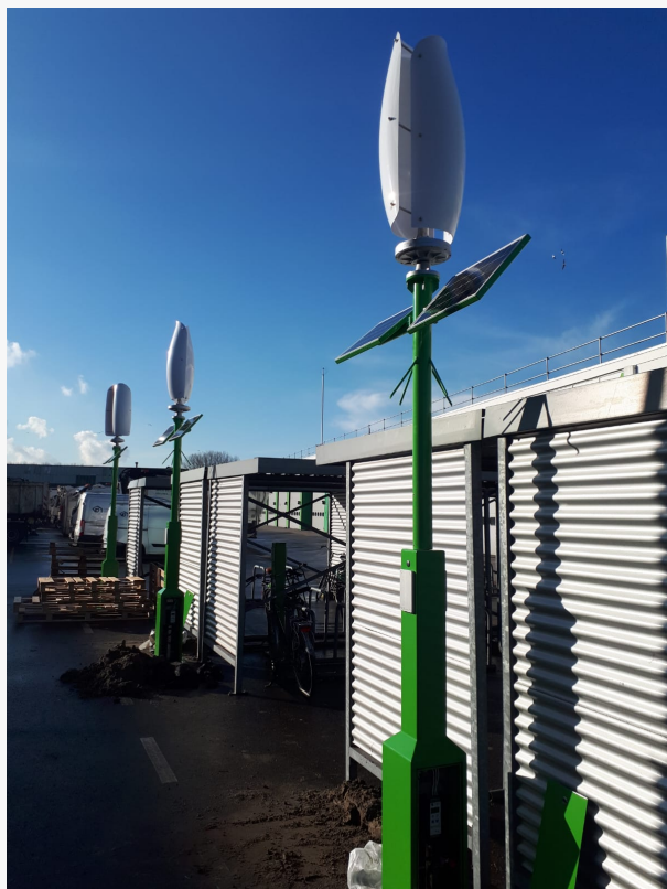
Wind and Solar E-bike Charging Poles
