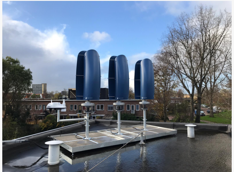
Three installed small size Wind Tulips
