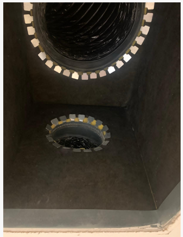
Dryer Vent Cleaning Service in Port St Lucie
