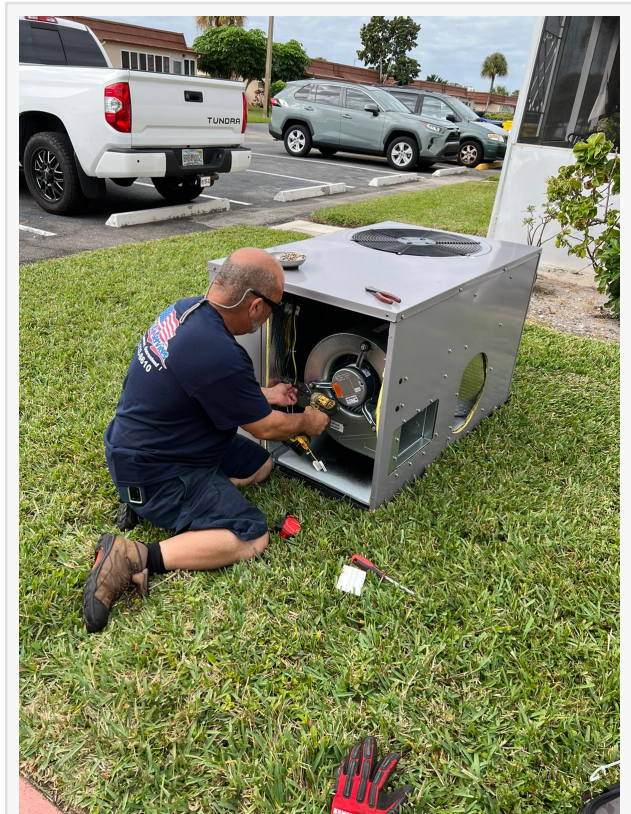
AC Repair Services
