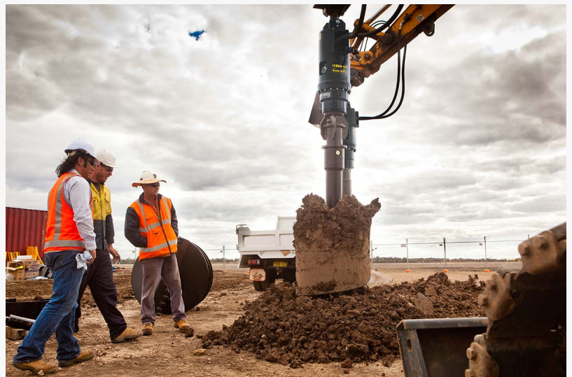
The Solaris-Auger Torque Earth Drill on an Excavator
