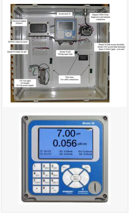
To ensure easy access and protect the equipment, KECO built all of the level, pH, and wireless equipment into a Saginaw 24" X 24" polycarbonate enclosure. This features a door and window, allowing operators to view the display without opening the door.
