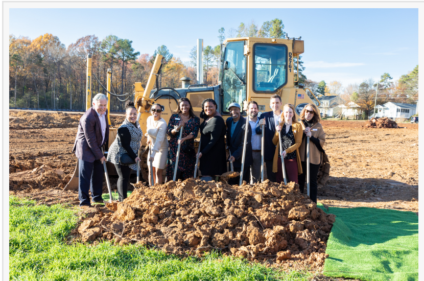
Community partners and developers break ground at the site of Historic Nathaniel Carr affordable homes for seniors.
