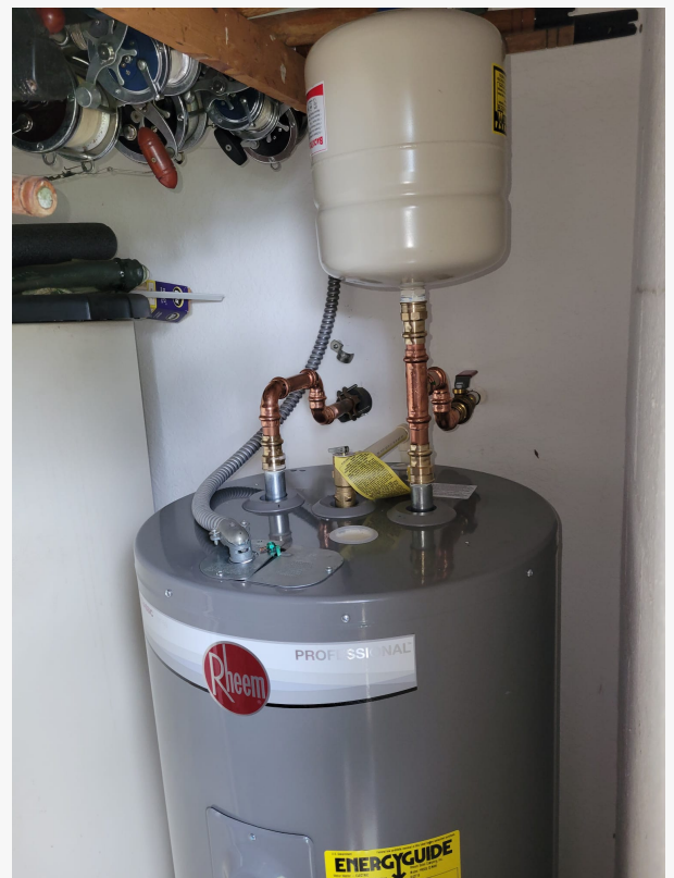
Water Heater Repair Services
