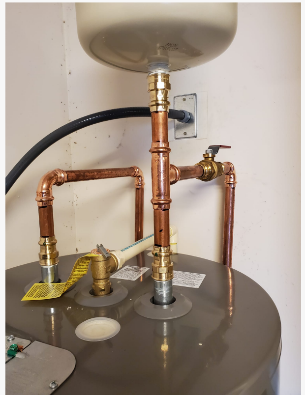
Water Heater Repair Saint Lucie County
