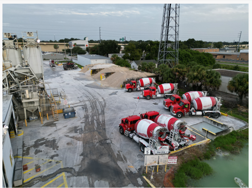
Kennedy Concrete plant Orlando, Florida.
