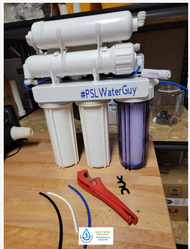
PSL Water Guy - Reverse Osmosis System Installation
