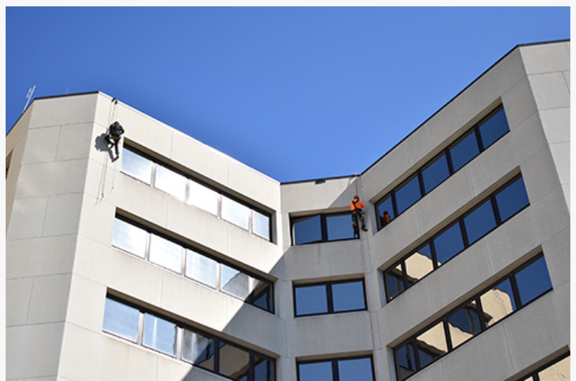
Get Bats Out rope tech performing a commercial bat removal project
