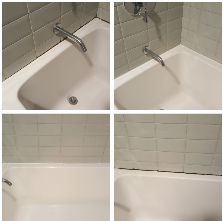
Before and After bathroom shower/tub grouting repair
