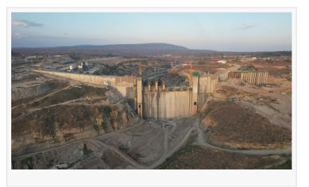
demolished the cofferdams upstream and downstream of the main dam, in parallel to ongoing installation works for the large Francis vertical turbines that are capable of producing annually approximately 6,307 gigawatt.hour of low-cost energy in Tanzania.
