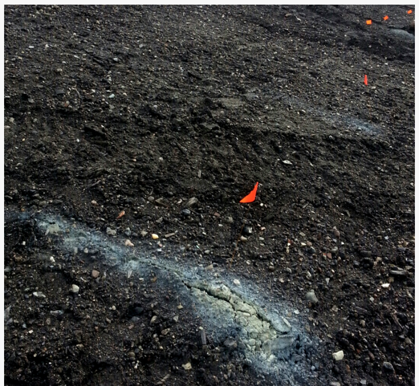
A "Scab" is where concentrated toxic landfill gas has denatured and destroyed cover soil and clay cap material. The gas pours out in high levels at these locations
