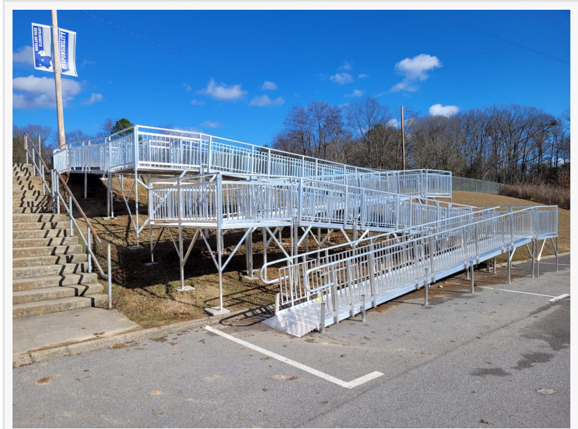
146 FT ADA-Complaint Commercial Ramp
