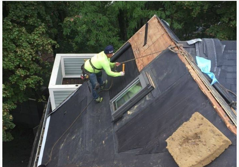
Worcester roofer completing a roof replacement on a home
