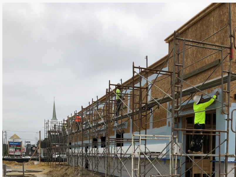
Whiteville Urgent Care groundbreaking + construction
