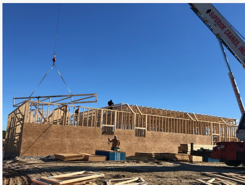
Williamston Urgent Care groundbreaking + construction
