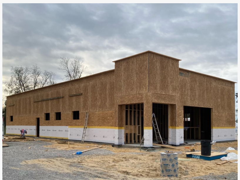
Elizabethtown Urgent Care groundbreaking + construction
