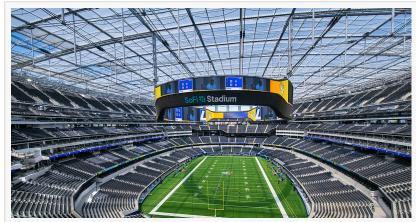
PFEIFER Structures America completed the monumental cable-net-supported ETFE roof for SoFi Stadium in Inglewood, California.
