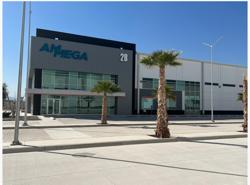
New Ammega facility in Torreon
