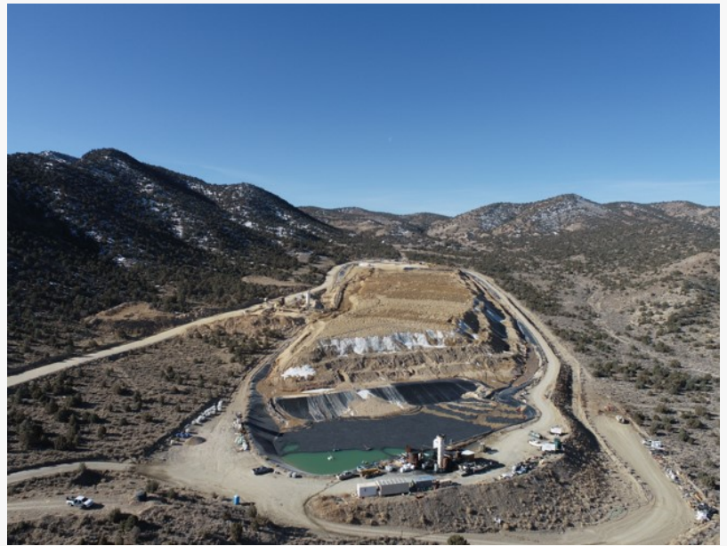
Desert Hawk Gold's existing two million ton capacity heap leach pad and processing facilities
